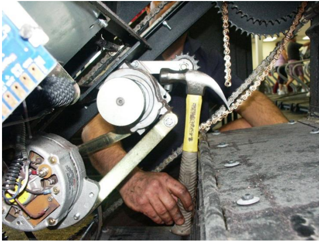
Figure 9. Placing the Hammer Between the Idler and Step
