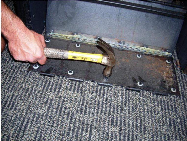
Figure 9. Installing New Push Nuts
